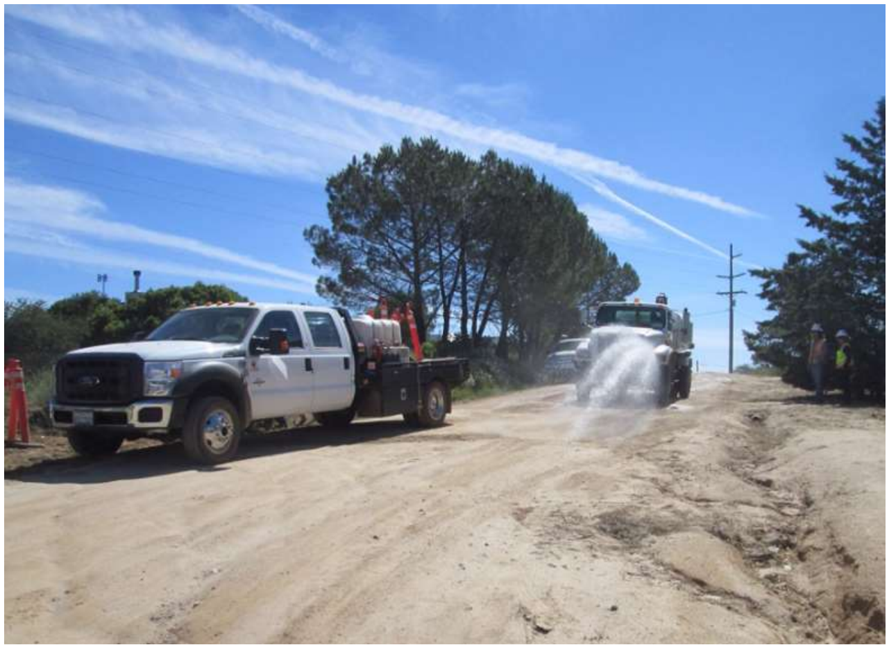
Photo 1: During conventional pole hole drilling at Z44263 (TL 6931), crews watered the access road for dust control in accordance with APM AIR-02.
